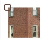
Brick veneer (original wood frame structure underneath)
